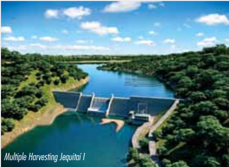
Belo Monte Hydroelectric Facility - Pimental Site
